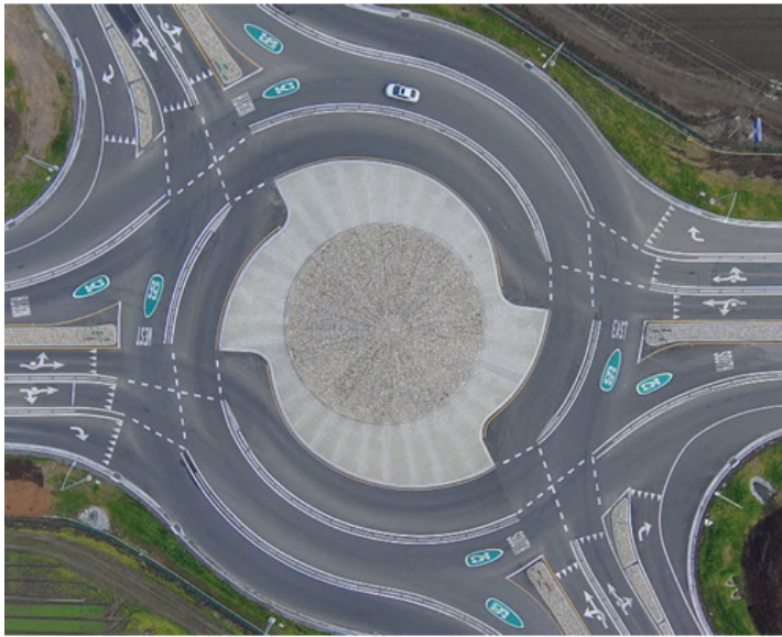
Figure 4. Overhead view of the pavement markings at the roundabout.
