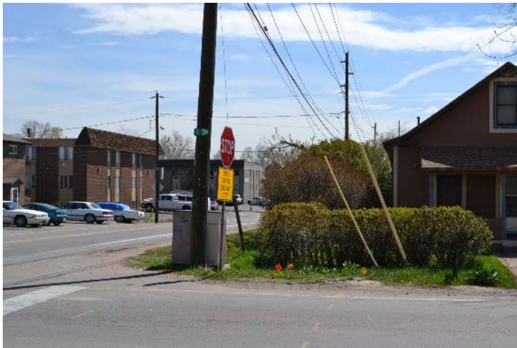
Poor Sight Distance at the Intersection
