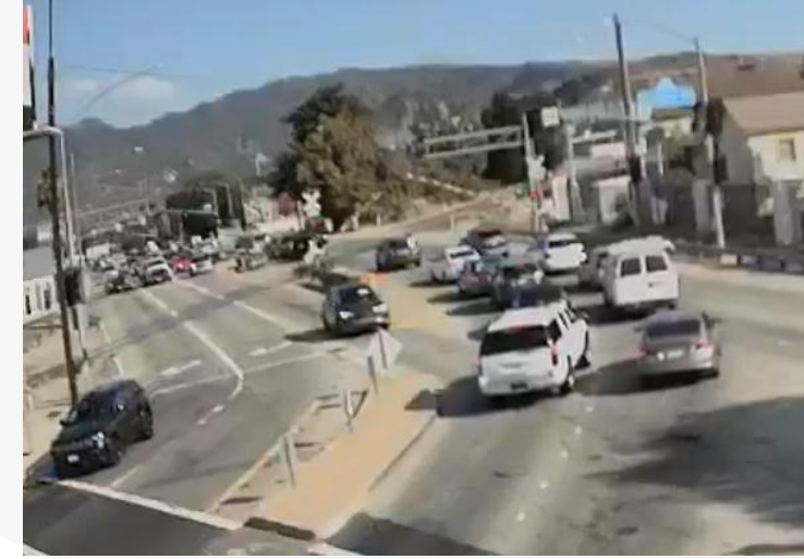
Eastbound Queue Spillback at Newhall Avenue Railroad Crossing
