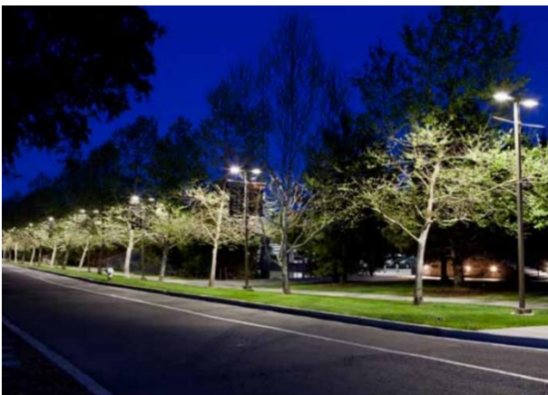
Network-controlled adaptive LED fixtures line Old Davis Road on the UC Davis campus.
