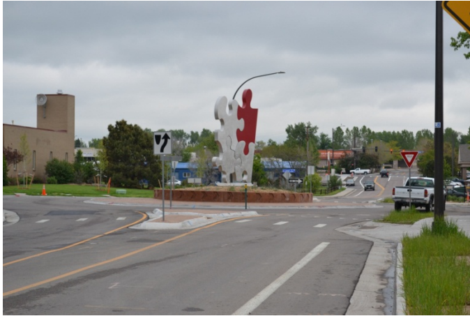
Newly Constructed Roundabout with Center Art Piece
