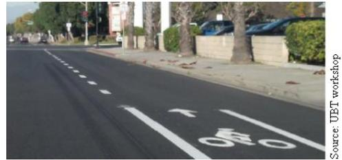
Figure 10: Right buffer dropped at intersection
