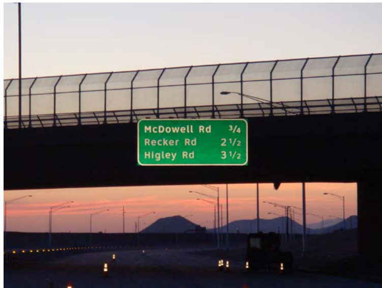
FIGURE 2 Typical Overhead Sign Location
