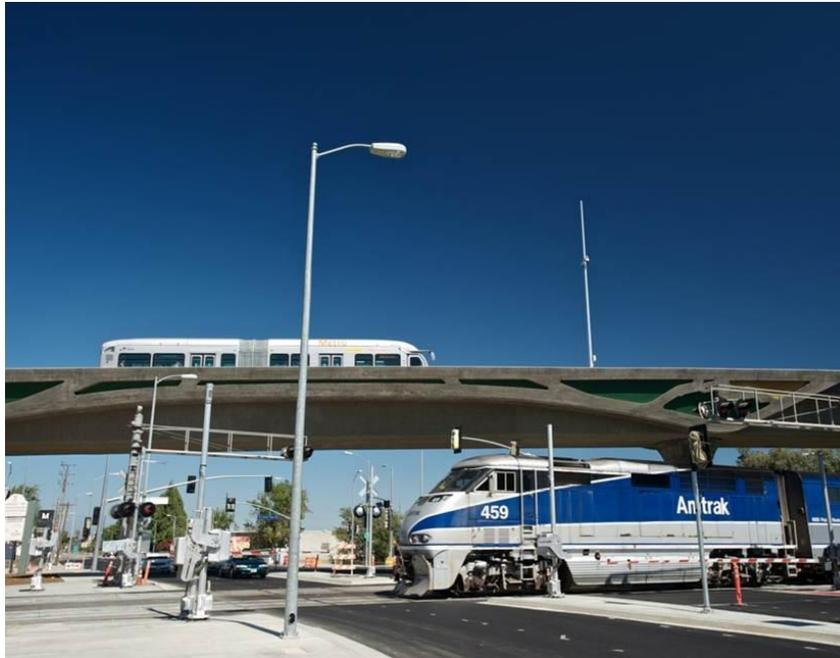
The preparation of the final design plans for the overcrossing required coordination and approval by Metrolink, the UP railroad and the California Public Utilities Commission (PUC). It was a complicated design process because the busway overcrossing crossed the tracks at an angle in a location where the railroad right of way was tight. The placement of the overcrossing support columns, the approach ramps and the at-grade bikeway/pedestrian
