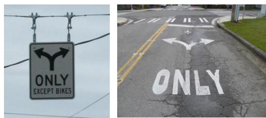
Figure 3. Turn Restriction Sign and Pavement Markings
