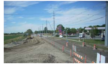
Grand Avenue roundabout (west approach)
