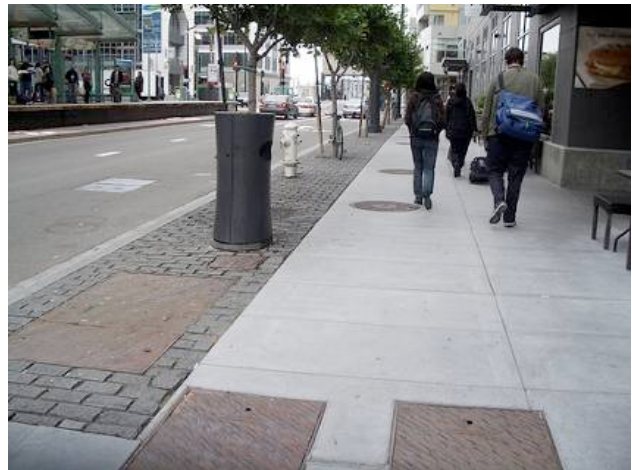
Figure 5 shows an example near 4th & King in San Francisco shows how textured pavement could be a potential solution to demarcate flex-space from the accessible path of travel. source: author photo
