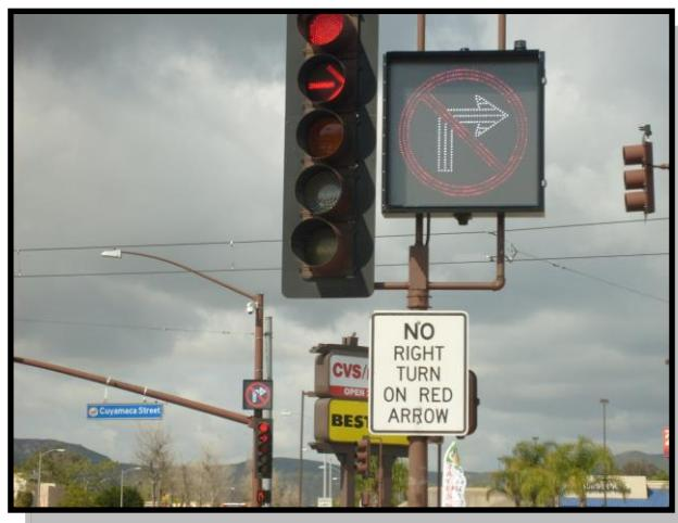
The sign is displayed only when trolley is detected in the system and the westbound through movement has the red to prevent conflict between the trolley and the westbound right turn movement. The sign is blank in the absence of trolleys so westbound movement can make right turns on red.
