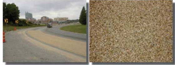
Application of Tyregrip® friction material on a curved ramp.
